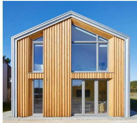
Ringmer Passivhaus, (Photo courtesy of Enhabit)
