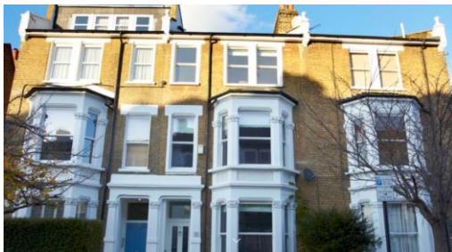
Lena Gardens – UK’s first Passivhaus Retrofit (Photo courtesy of Kingspan)
